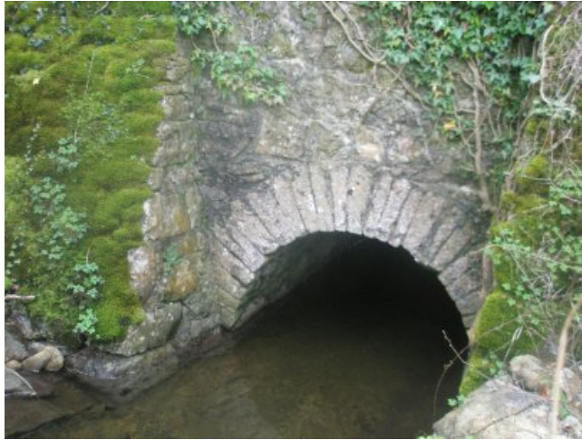
Fig. D: Jasper's Bridge. Photo: Declan Barron
